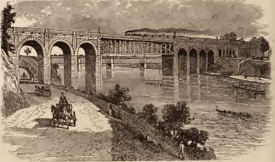
CONNECTING RAILROAD BRIDGE, FAIRMOUNT PARK.
